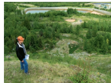
Overview of the Samatosum surge pond and treatment plant.
