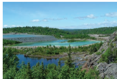
Overview of the water-covered Winston Lake tailings facility.
