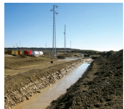
Storm water diversion structure around the Las Cruces open pit.
