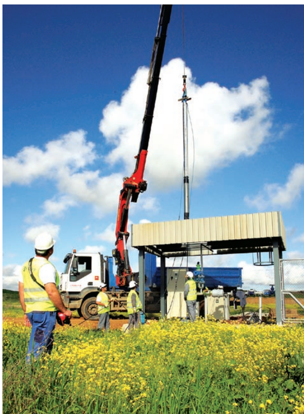
Maintenance of a dewatering well.
