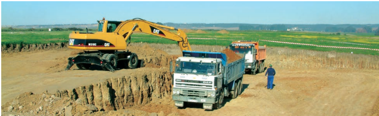
Beginning of site preparation at Las Cruces.
