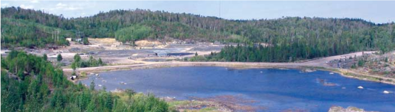
Polishing pond at the closed Winston Lake property. The pond assists in improving the site drainage water quality prior to release to the adjacent creek.
