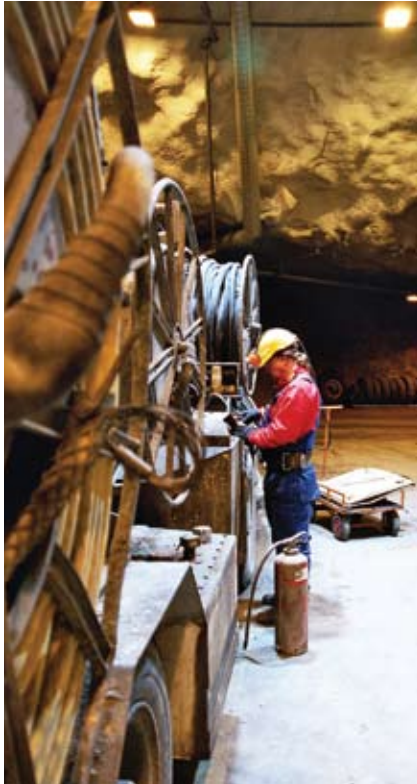
Underground equipment inspection and maintenance at Pyhäsalmi. Preventive maintenance helps us improve our safety, environmental and production performance.
