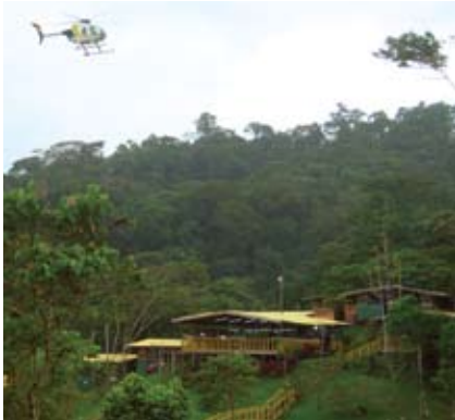
The core logging and sampling building at Petaquilla's Colina Camp.
