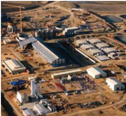
Aerial view of the plant construction at Las Cruces.
