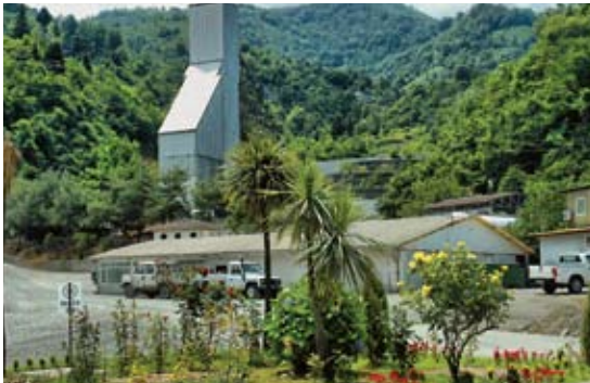
Runoff management within the steep terrain at Çayeli can prove difficult. Çayeli is assessing measures that will improve runoff management and help reduce its consumption of fresh water from the aquifer and river.
