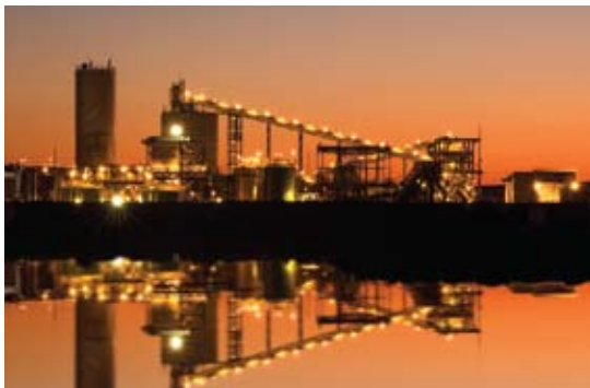
The Las Cruces processing facility was ready for commissioning at the end of the year.
