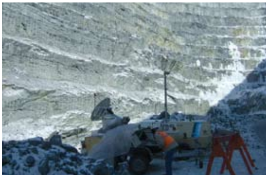
Troilus pit wall continuous stability monitoring during the final months of mining. The radar unit detects millimetre scale movements during its eight minute scan of the entire pit wall.
